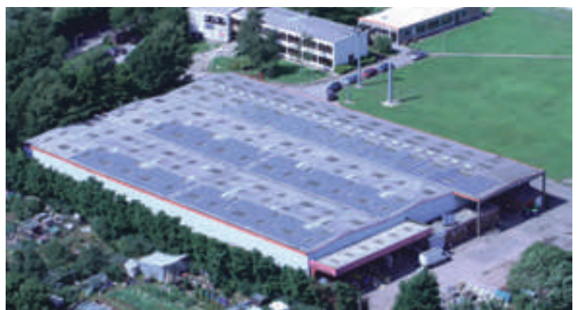
Burley's factory in Oakham with 200kW of solar panels.
