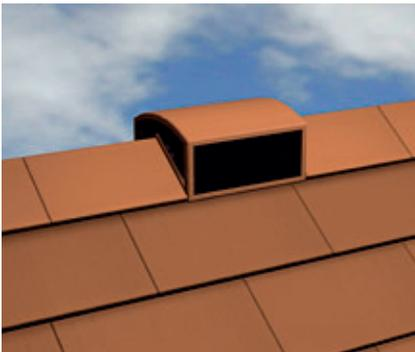
Modern houses generally later than 1960 often have a pre-cast concrete chimney system, identifiable by a rectangular box section flue and a terminal, as illustrated in the picture above.
