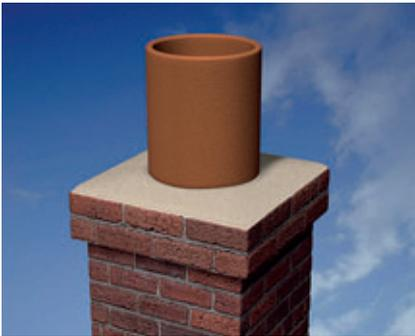
Commonly in older houses, earlier than 1960. The Class 1 chimney is identifiable by 7" (180mm) or greater diameter flue. The existing chimney must be structurally sound, please check before the installation of a new fireplace.
